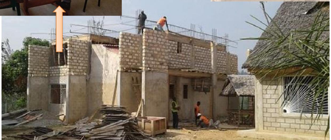
Hanze House: Below: Under construction. On top: In use!
